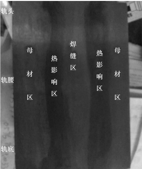
图 1 钢轨焊接接头的纵向剖面宏观形貌 Fig. 1 Macro profile of longitudinal cross-section of rail welded joint
